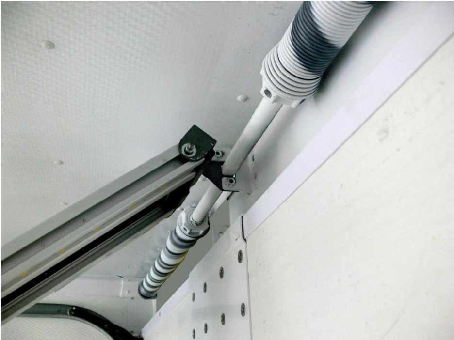
Connecting the track to the header
