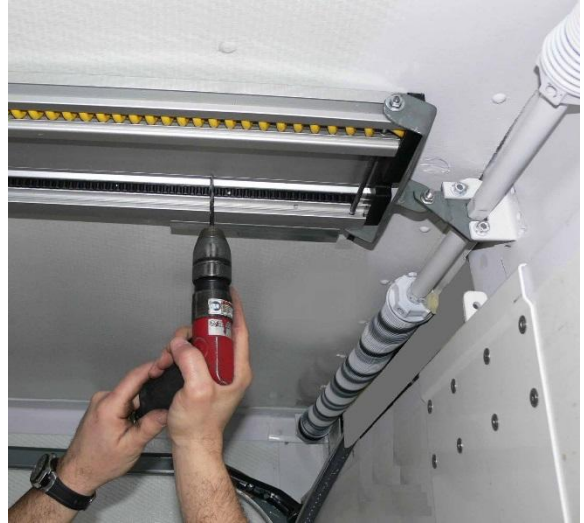
Drilling the roof bows
