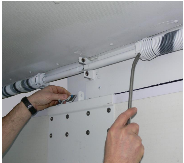
Figure 8 – Adjusting the door balancer
